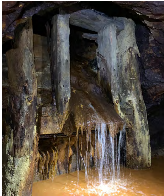
Drainage level ore chute
