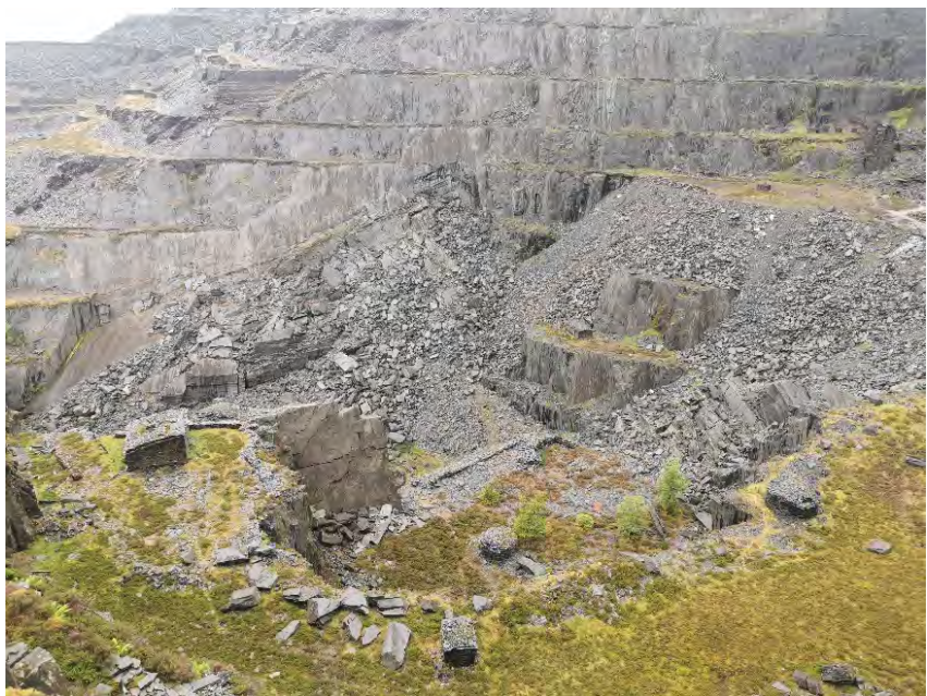
Looking down into the quarry- notice the remains
