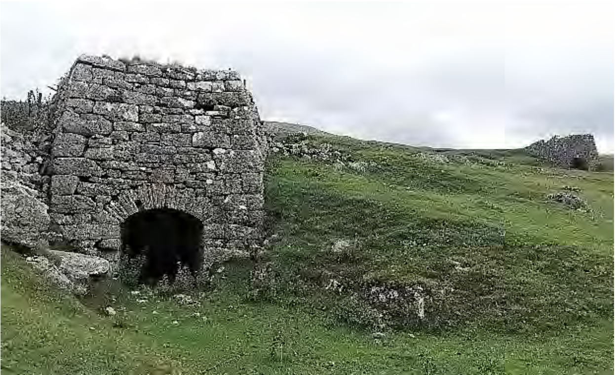
The two line kilns.
