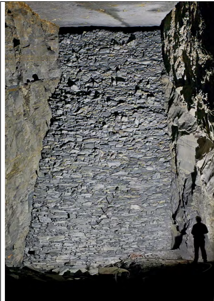
Pack wall in Chamber E31OV
