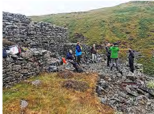
Crusher and ore bins
