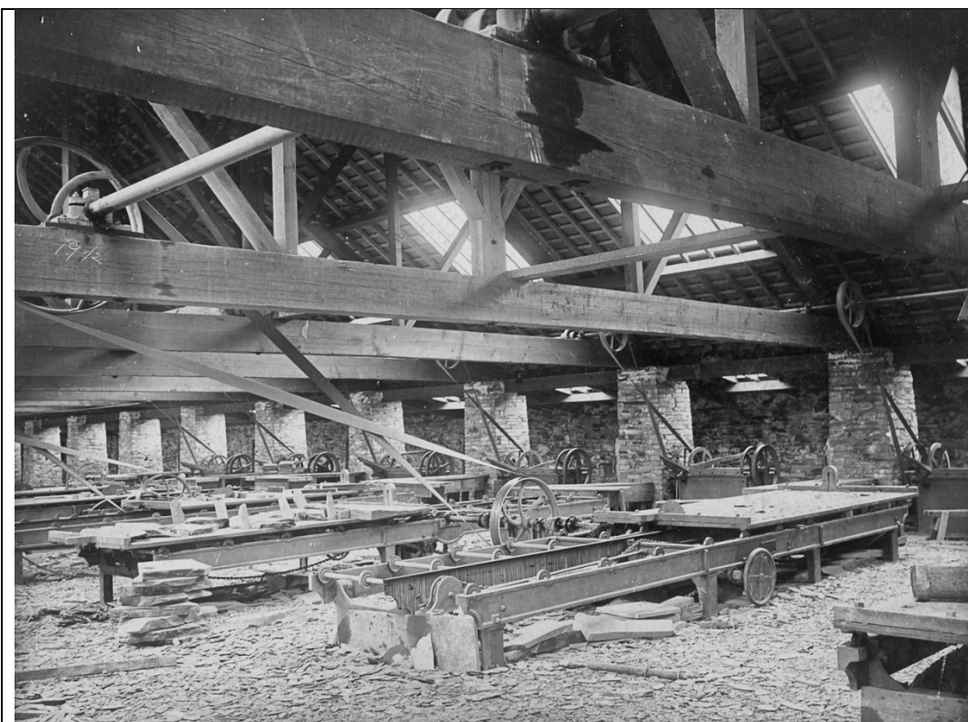
General view inside the Mill shortly after completion.
