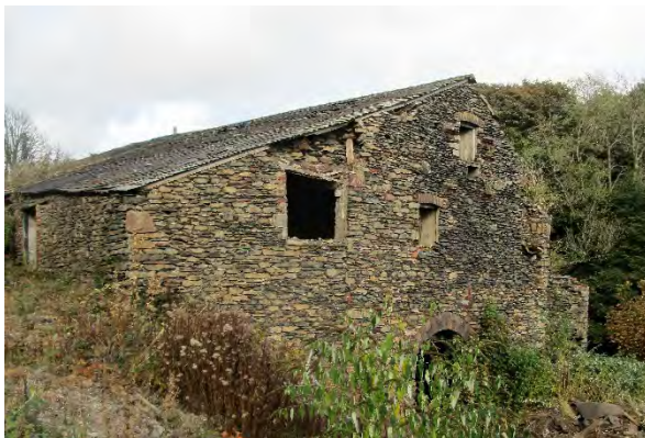
The pug mill, site of a forge which existed prior to 1711.
