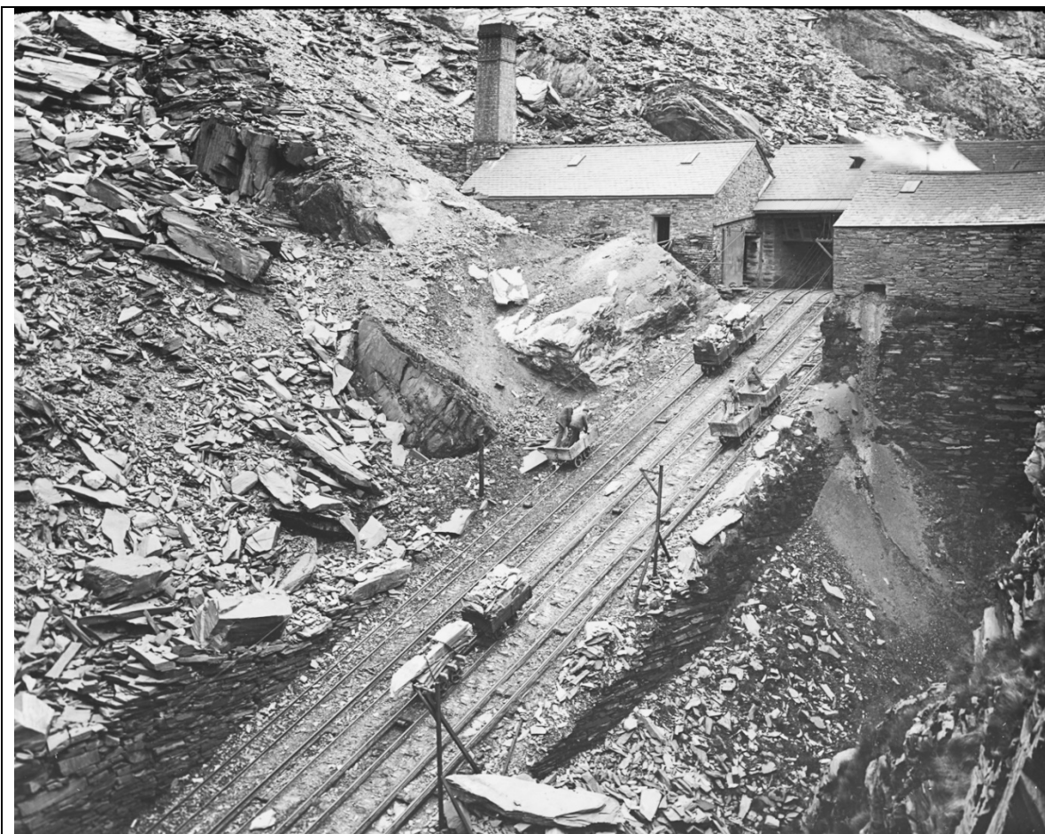
Back vein incline, the principal route by which waste and rock was brought out of the mine.
