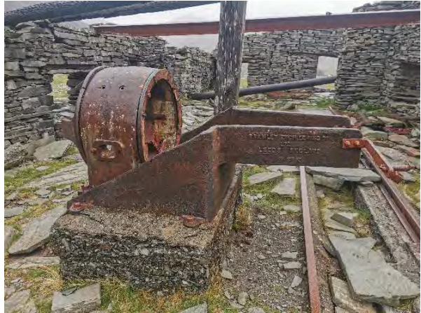
Inside the saw shed
