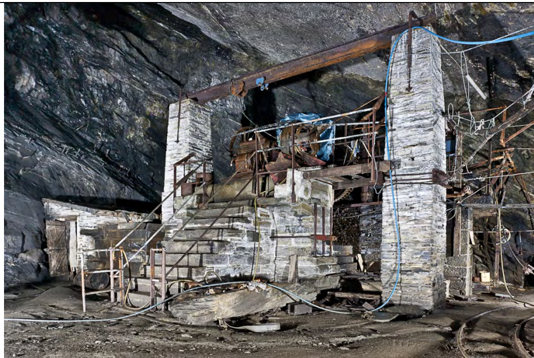
Chamber 8 old vein showing incline winder. This was initially steam powered but then converted to electricity at 500V dc.
