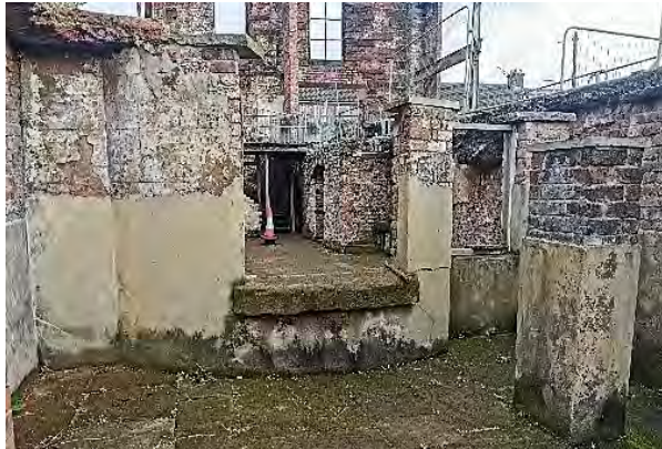
Bay window of the house
