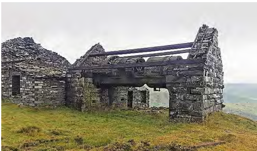
Remains of one of the many incline winders
