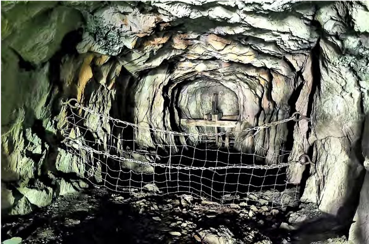
Top of the Old Engine shaft
