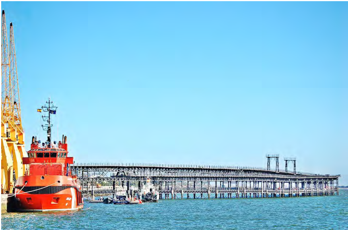
Huelva Pier came into operation 1876, photo shows the three levels. The bottom level housed coal bunkers for imported Welsh coal, the middle level was from where the waggons discharged copper ore into ships holds, for export to Cwm Avon Copper Works near Port Talbot.
