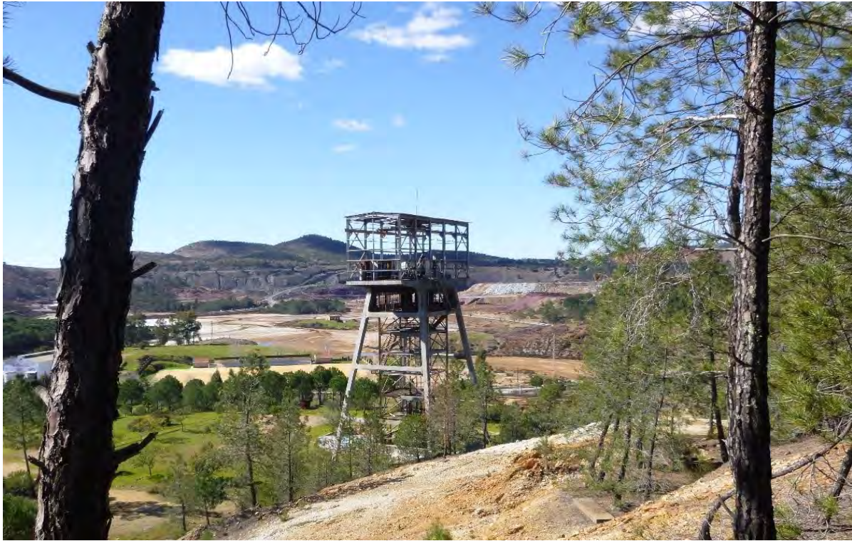
Pozzo Rotilio, this was the last headstock to be built in the mining basin 1960.
