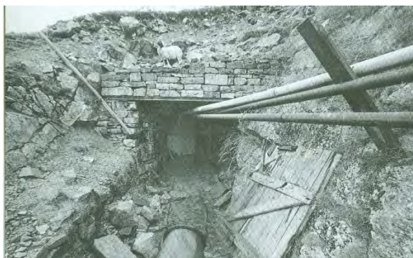
Carrock Mine entrance just after closure
