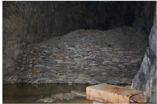
Slate Close head in Tilberthwaite Horse Crag Level used a dump for the spoil from the first fall- before and after.
